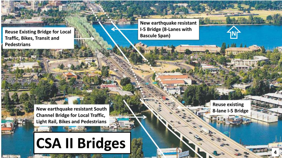
This slide shows a ground-level view of the bridges shown in the previous slide. Note that the new freeway bridge would diverge northbound from the current south channel bridge as it crosses Hayden Island. This new bridge is designed to carry primarily long-distance interstate traffic between Oregon and Washington, including most of the freight traffic.
